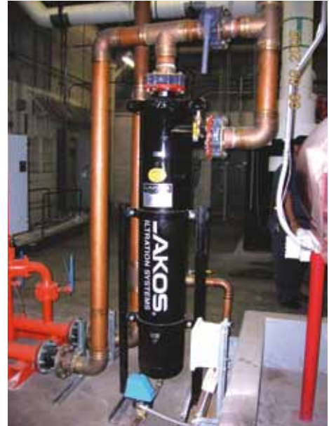
HTX used to prevent sand from entering toilets and other water supplies at large Convention Center in Florida
