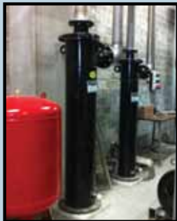
Cleaning chilled water, Axima Belgium
